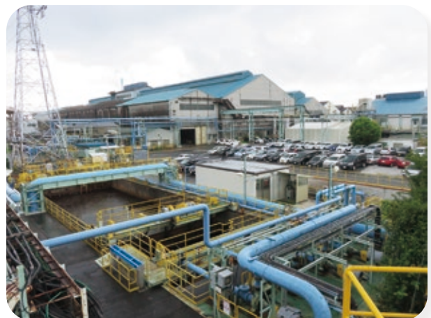
Wastewater treatment at the Hoshizaki Plant
