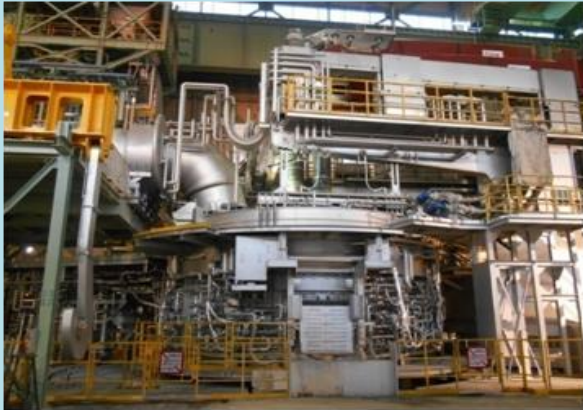
[1] Electric furnace with a rotating body (150 t) Installed in 2014
